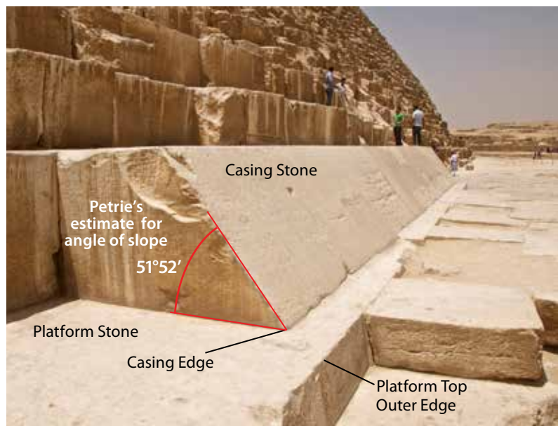
Casing and Platform Stones. Near the corner of the north side the angled casing stones sit upon platform stones. The lower, outer edge of the casing and the top, outer edge of the platform provide the best places to measure the Pyramid's lines. Petrie estimated the angle of the casing slope to be 51° 52 minutes ± 2 minutes. Photo by Mark Lehner.
